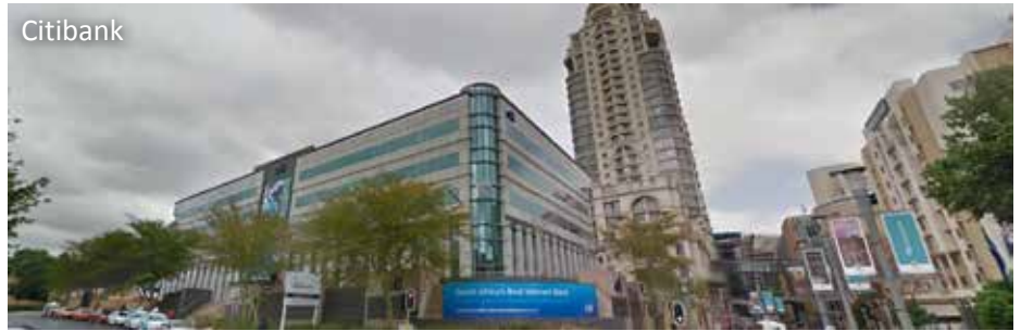
Fourways Mall development
